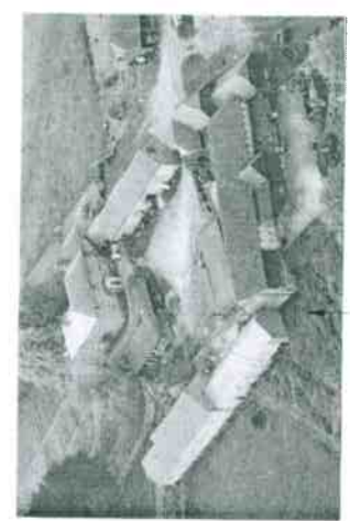
End bay of barn and central passage to be retained. Existing structure removed under Planning Application Ref: 17/02476/1 & 17/02476/2.
